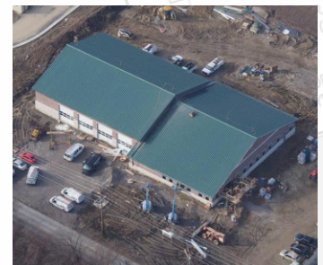
Aerial view of the in-progress station
