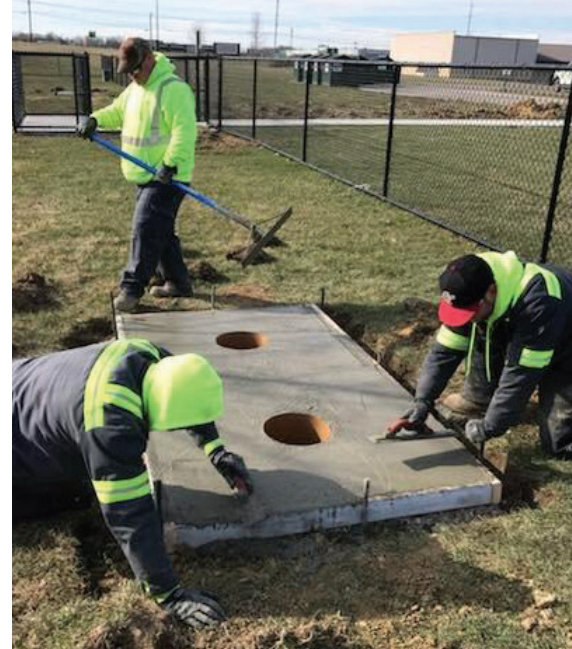
Service Department makes repairs to Holly's Dog Park
